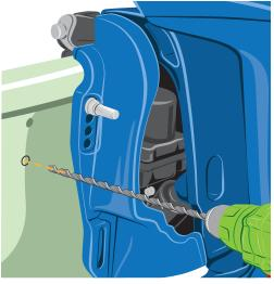
**1d.** Remove the base plate and drill your second 1/2" hole where you marked.
