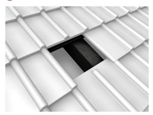
The rafters, on which the roof fasteners are to be mounted, must be exposed. The height of the roof fastener must be checked and adjusted if necessary.
