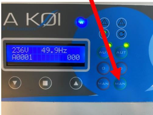
If you keep this button pressed, the pond pump will stop and the motor and rinse pump will be activated. When you release it, the system will turn off. Then press the AUT buttons again (green light will turn on again) to reactivate the system (pond pump will turn on again).
