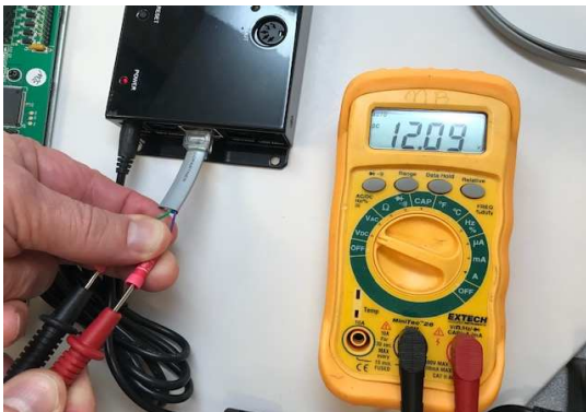
Checking voltage out of CPU
