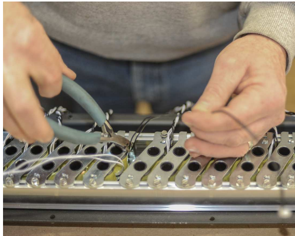
Illustration 123 - Cutting wires on unused solenoids.
