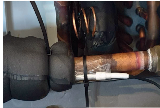
Place sensor on copper pipe
