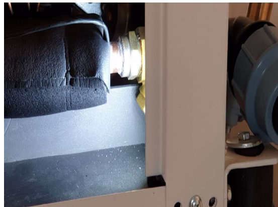
Move the isolation sleeve back to cover the sensor and route the cable to the controller.
