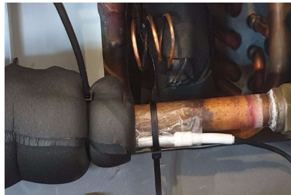
Place sensor on copper pipe
