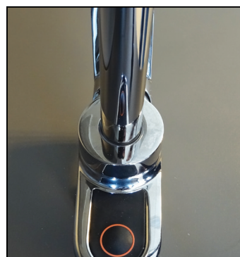
Step 6 Tighten the nut firmly on the tap housing so that all play is gone.
