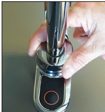
Step 1 Loosen the nut that secures the tap spout on the tap body.
