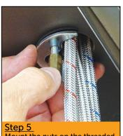
Mount the nuts on the threaded ends, use the supplied box spanner to firmly secure the tap to the worktop.
