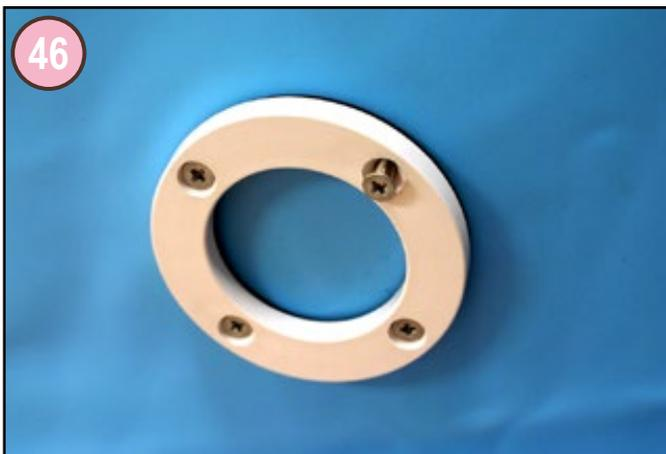
Screw the flange (fitted with its gasket) into place using the countersunk SS screws M5x16 from the pool fitting skin pack. Tighten the screws alternately to ensure a leaktight fit. Hand tighten, over tightening could damage the flange.
