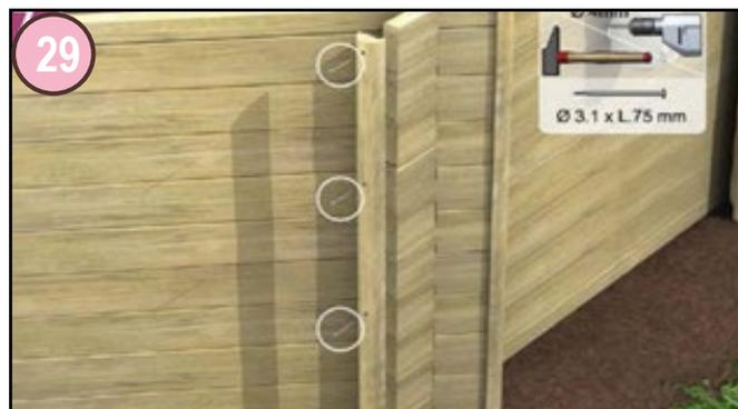
Mount a decorative profile (type H) on the end of each wall using nails (3.1x75mm) inserted through evenly spaced holes pre-drilled along the axis of the profile.
