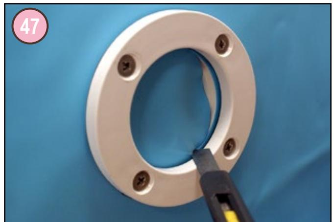
Using a Stanley knife, carefully cut the liner following the inside of the return fitting.
