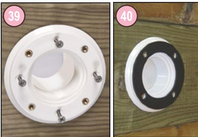
From the pool side, insert return fitting throughwall flange (pool fitting pack) into the opening in the machined slats.
