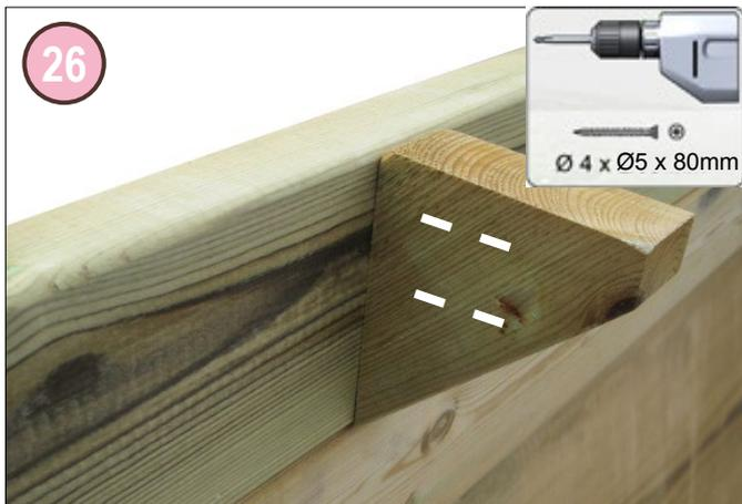
The wooden corbels will support the coping that will be mounted after the pool is filled. Pre-drill the wall from inside the pool then attach each wooden bracket (type L) using 2 screws (5x80mm sachet R) taking care to position them flush with the top of the structure. Remove any splinters that may have been raised during this process.
