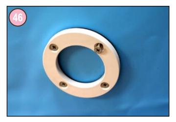
Screw the flange (fitted with its gasket) into place using the countersunk SS screws M5x16 from the pool fitting skin pack. Tighten the screws alternately to ensure a leaktight fit. Hand tighten, over tightening could damage the flange.
