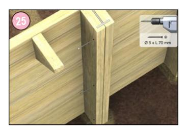
Working from the outside, fasten the cradle's vertical posts (pre-drilled) onto the wooden walls using 6x30mm screws from bag S. Check their verticality. Position two decorative profiles (Q) on either side of each post and fasten them together using 3 5x70 screws (bag S) as shown.
