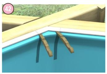
Place the liner in the centre of the pool and unfold it. When it is unfolded, the liner will form either an octagon, an elongated octagon or a hexagon on the ground, depending on the pool model. Line the corners up with the corners of the pool structure. Working in bare feet from inside the pool, fit the liner lip into the liner locking track, continue around the pool.
