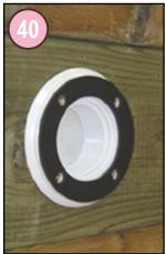
From the pool side, insert return fitting throughwall flange (pool fitting pack) into the opening in the machined slats.
