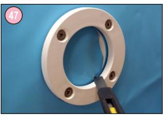
Using a Stanley knife, carefully cut the liner following the inside of the return fitting.
