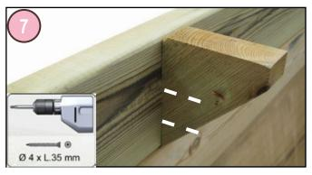
The corbels will support the coping that will be mounted after the pool is filled. Pre-drill the wall from inside the pool then attach each wooden bracket (type L) using 2 screws (5x100mm sachet J) taking care to position them flush with the top of the structure. Remove any splinters that may have been raised during this process.
