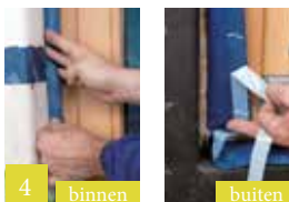
4 Band rondom in de dagkant vastkleven
