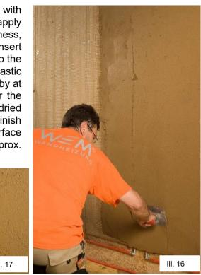
A single plaster coat must not exceed a thickness of 10 mm!
