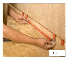
When bending the pipes, observe a minimum bending radius of 80 mm, when bending by hand, and of 64 mm, when using a spiral spring!
