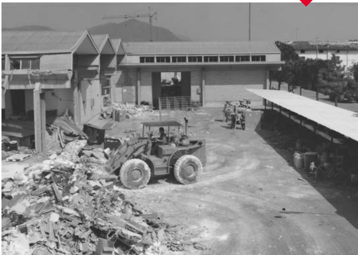
Ledraplastic plant during post-earthquake reconstruction (1976)
