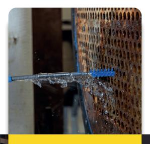
This operator is cleaning a watercooled chiller. The (blue) flexible shaft is used to rotate the brush inside the tube to remove deposits. At the same time, low pressure water flows through the shaft to flush out loosened deposits, cool the brush, and shaft core.
