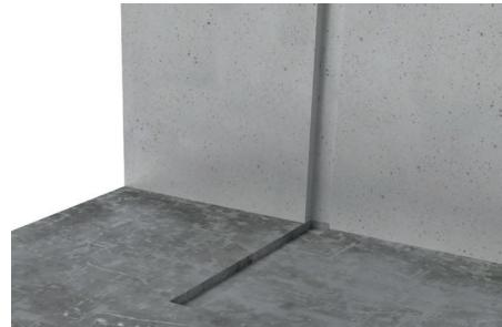
2 conduits have to be installed; One for the sensor and the other for the power cable from mat. Do not run the power cable and sensor cable through the same conduit. Cut a groove in the floor for the floor sensor pipe (2 cm deep).
