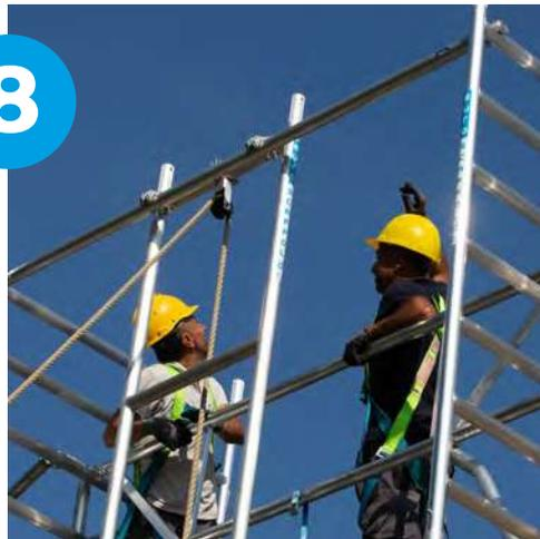
Mount the last part when the desired height is reached and connect it with the securing clips. Then connect the pulley to the upper lift frame. Make sure that the line is pulled through the top pulley before mounting the top lift frame.
