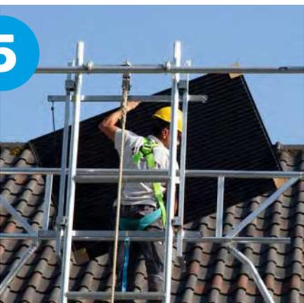
Lift the panel over the handrail on the platform.
