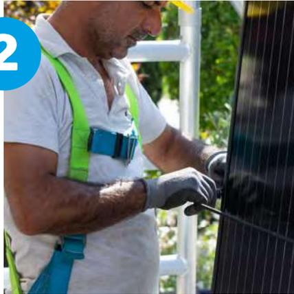
Secure the panel on the carriage with the elastic tensioner.
