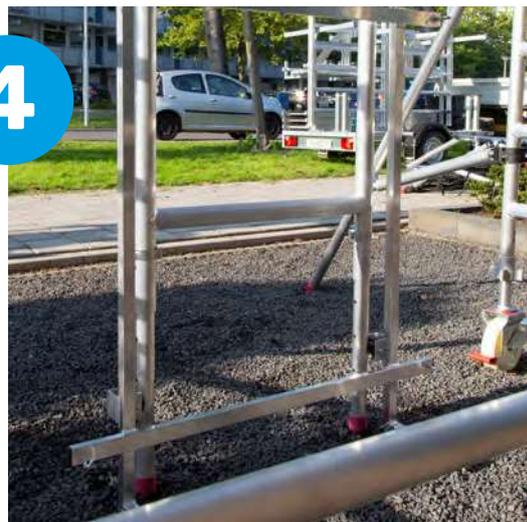
Slide the carriage onto the base lift frame
