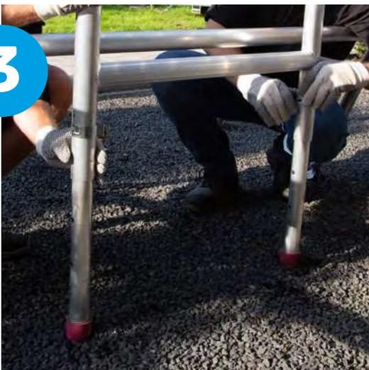
Mount the levelling legs into the base lift frame.
