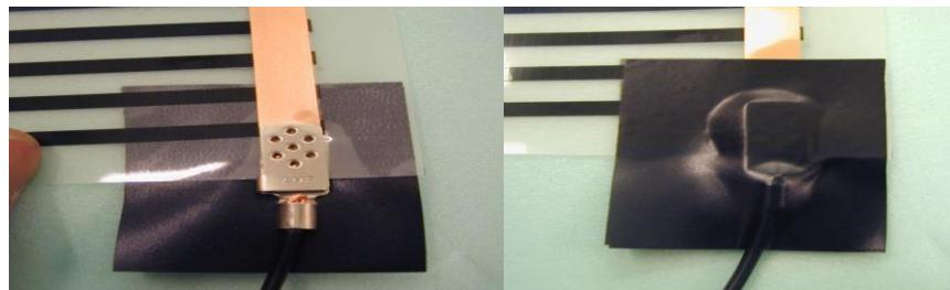
**After installation. NOTE :** always insulate the crimp connectors. Cut 2 pieces of insulation tape and stick them over the crimp connectors on both sides. The tape must be placed well over the end of the crimp connector, at least 5mm. The end of the underfloor heating foil should also be insulated with insulation tape.
