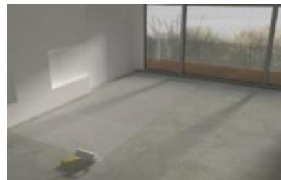
Make the surface clean and level where the foil will be placed. It is mandatory to place insulation under the underfloor heating foil. Quality Heating has various insulation options. Go to the webshop or contact customer service. If you have a damp subfloor, use the FastHeat floor primer as a primer.
