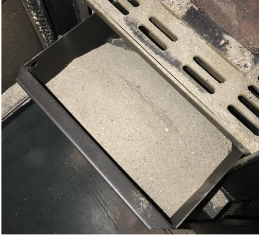
Example of a dirty ash pan Example of a clean bottom
