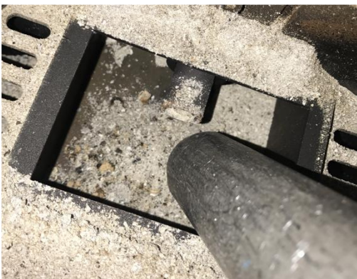
Example of a dirty soil
