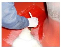
Apply an evenly <u>thin</u> layer of "LUWIREP PU- and metal primer" on the roughened area and let primer dry for approx. 20 minutes\*.
