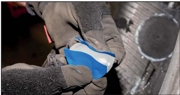
14. Bend the repair back and push up on the edges of the repair with your fingers to break the perforation on the protective poly on the back of the repair. Partially remove the poly, exposing the middle portion of the repair.
