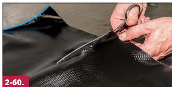
Cut a piece of cushion gum to the size of the buffed surface and over buffed area on the inner liner.
