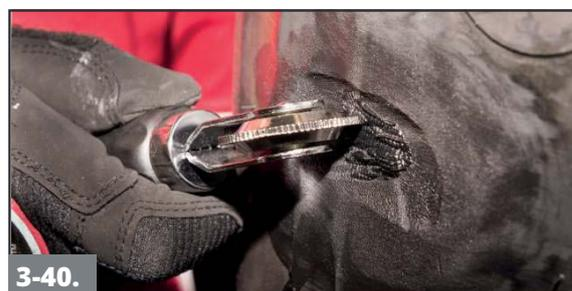
**3-40.** Use a Skive packing tool (#985 or #986) or a stitcher to pack the rubber into the injury channel and to remove trapped air.
