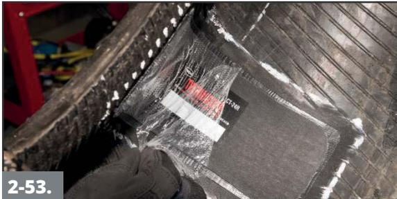
Remove the clear poly from the top of the repair unit and inspect the repair unit for trapped air. If trapped air is found, stitch the repair unit again.
