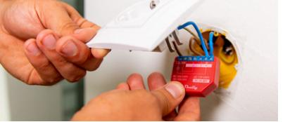
If you are using DC power supply, connect the wires as shown on **fig. 2**. Connect the load to the O terminal of the Device and the DC+ wire. Connect the GND wire to a L terminal of the Device.
