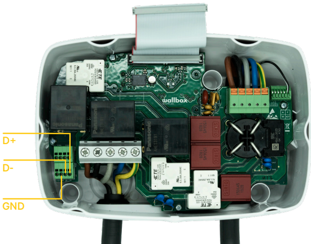
Fig. A1.6 Kabelinstallation i en Wallbox Commander 2
