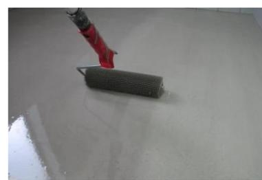
Levelling of the surface with a spiked roller
