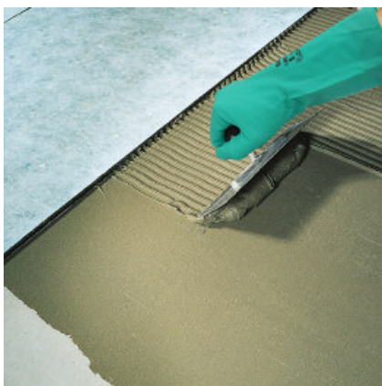
1. PCI Flexmörtel, PCI FLEXMÖRTEL S1 RAPID, PCI Nanolight of PCI Nanoflott Light opkammen.
