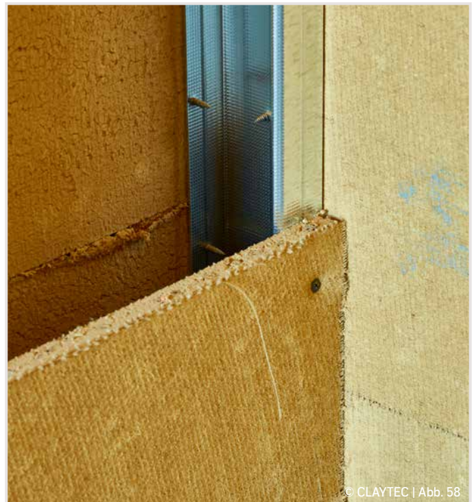
Detail inside corner
