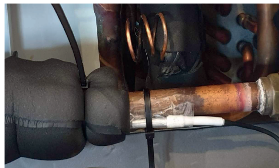
Place sensor on copper pipe
