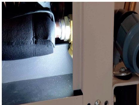
Move isolation back as far as possible
