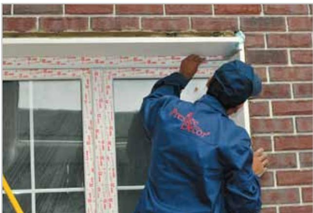
7. Check the correctness of slope angle towards the window plane using set square.
