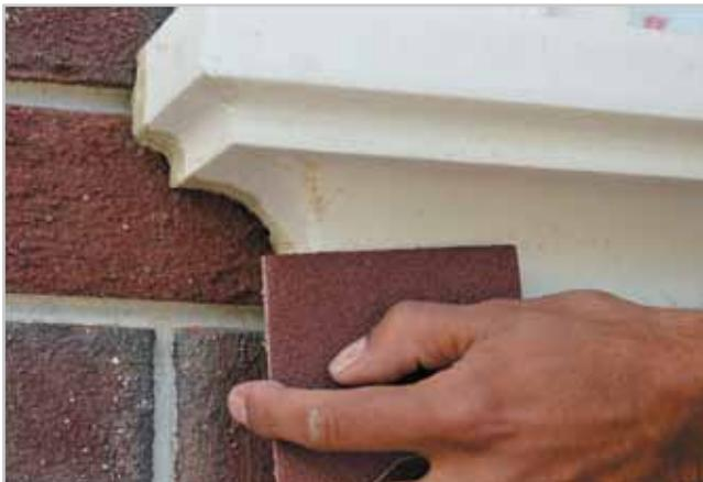
17. After thorough drying of the DarMix decorative and restoration mixture, smooth the joints and the renovated places with sand paper.
