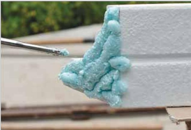
13. The fixfoam roller with about 15 mm in diameter must be applied on the whole surface of joint place of the element. Avoid cavities when applying.
