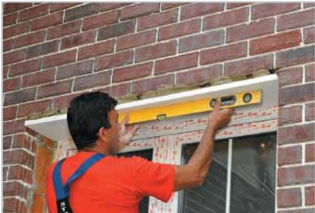
5. Check the horizontal position of the attached element using the measuring level.
