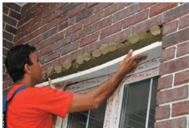
4. Press the element manually with the adhesive mass to the supporting surface. Continue pressing until the whole adhesive mass makes solid contact with the supporting surface.
