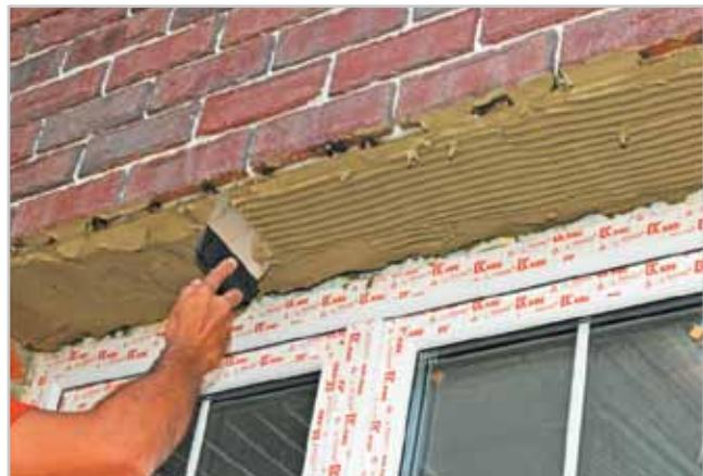
2. Apply the adhesive mixture to the supporting surface of the building. When applying the mixture the grooves from the filling knife should be along the processed surface.
