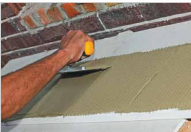
3. Prepare the slope element for installation. Apply the adhesive mixture to the joint place of the element with the supporting surface. When applying the mixture, the grooves from the filling knife must be perpendicular to the grooves of the supporting surface.
