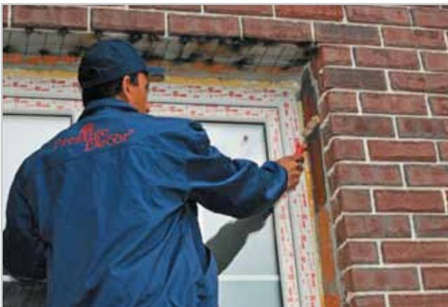
1. Remove any cement mortar, salt efflorescence, mould, dust and other pollutions from the supporting surface. Apply facade primer.
