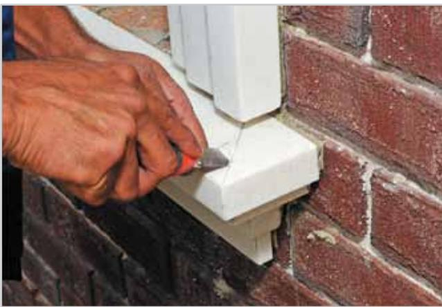
15. Divide all joint welds on the mounted items, leaving 2mm in width and deep from the top edge of the surface, to apply the DarMix decorative and restoration mixture.
