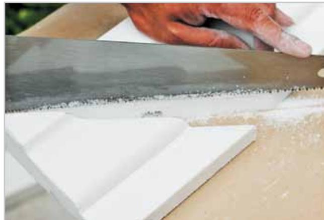
10. Cut the element with handsaw to the required size and configuration.
