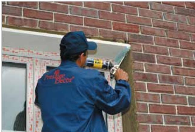
6. Apply fixfoam to the joint places of the elements. The joints are made with the fixfoam seam thickness of 2-2,5 mm. When applying fixfoam, consider the setting time, specified by the manufacturer on the balloon.
