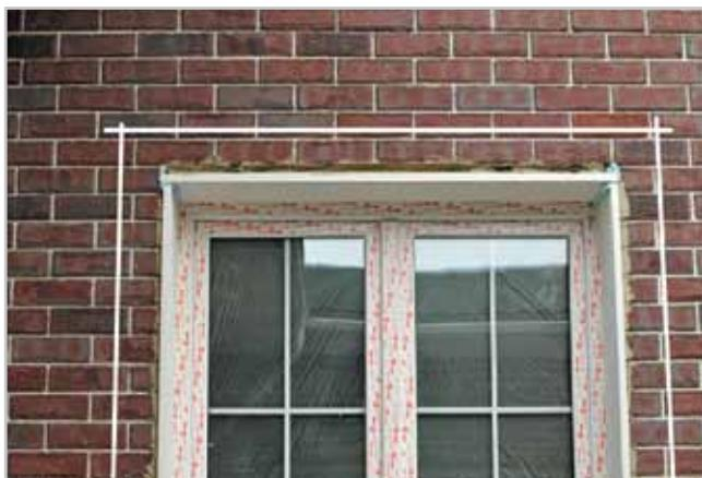
8. Make markings of the wall to attach the architraves using a chalkline.
