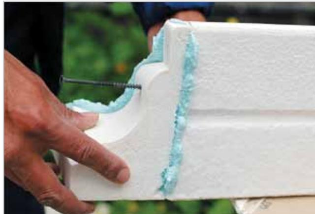
14. Fix the adherent elements carefully screwed in.
