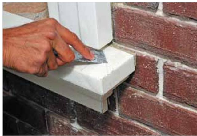
16. Cover the ready joint places with the DarMix decorative and restoration mixture using a filling knife, densely pushing the mixture into the weld.
