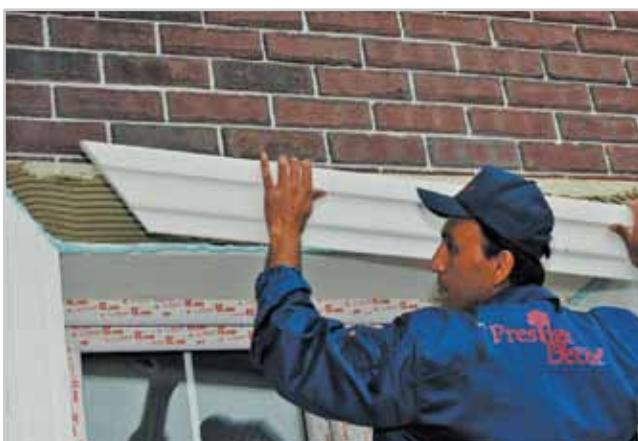
11. Stick down the mating surfaces of the details with painter's tape. Apply the adhesive mixture to the joint place of the element with the supporting surface. After removing the painter's tape, apply fixfoam to the joint place of details.
