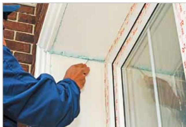
12. After thorough drying, cut down the excesses of the dried fixfoam. If cavities are detected, re-coat with fixfoam, wait until the surface is completely dry, and if required, cut down the excesses once more.
