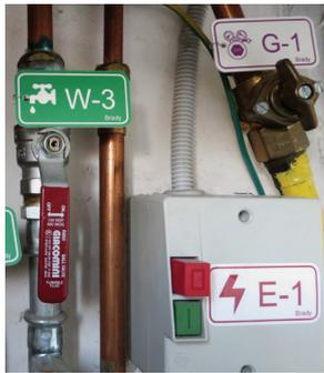
Energy source tags can be used to mark your facility's points of control for energy sources. These tags help make the lockout process quicker, safer and easier.
