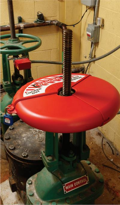
Brady's collapsible gate valve design provides secure lockout for a wider range of valves, with the use of fewer devices. These covers easily rotate around valve handles to the fully engaged position, while also folding into smaller sizes for easy storage on maintenance carts and in lockout kits.
