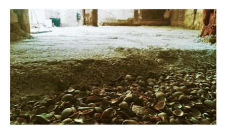
A floor build up on bare soil is also possible with CaNaDry. Place 25-30cm of shells directly on the soil and place the CaNaDry directly on the shells following the instructions above.
