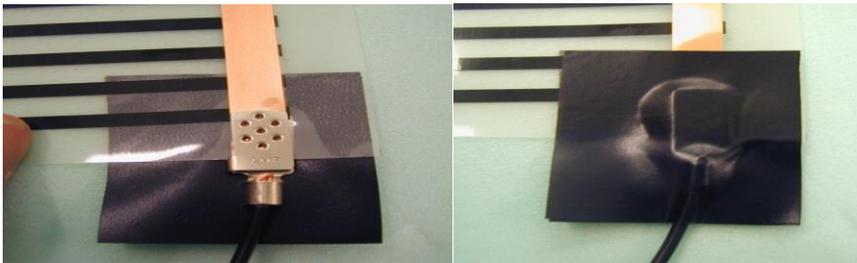
**After installation CAUTION:** Always insulate the shrink connectors by cutting 2 pieces of insulating tape and sticking them on both sides over the shrink connectors. The tape must be fixed at least 5 mm over the end of the shrink connector. The end of the underfloor heating foil must also be insulated with insulation tape.
