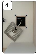
Connect the CAT6 cable and slide it into the venting shaft.
