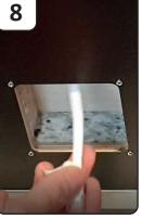
Grab the CAT6 cable and connect it to the connecting on the dish.
