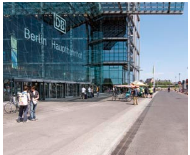
Main station Berlin, Germany
