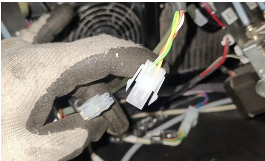
Figure 7 Disconnecting extruder cable
