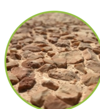
Deep exposure. Exposure depth approx. 4 mm
