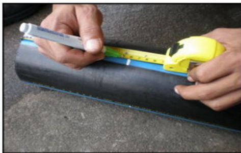
4. Mark the insertion depth on the pipe according to the 'Insertion table'.
