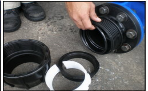
3. Assembly of the set components before pipe insertion.
