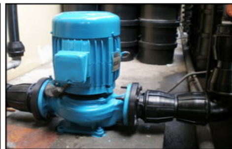
7. A Flange Adaptor tightened to a stem gate valve or onto a vertical in-line pump.
