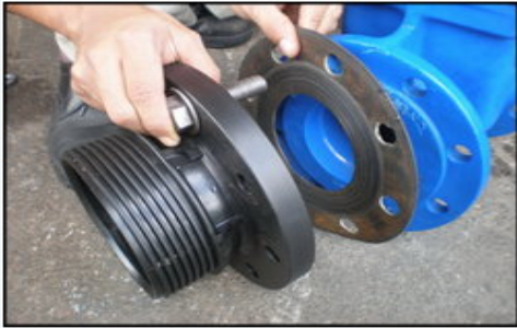
1. Dismantle the Flange Adaptor's components before fixing onto stem gate valve.
