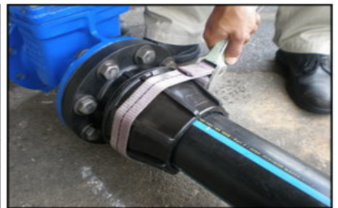
6. The locking nut can be tightly fastened by hand, with a tool or a strap wrench.
