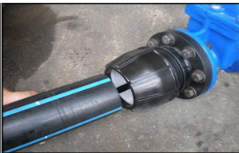
5. Loosen the locking nut by one or two threads then insert the pipe into the fitting to the correct depth according to the 'Insertion table'.
