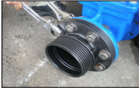
2. Tighten all bolts, nuts and washers onto the stem gate valve.
